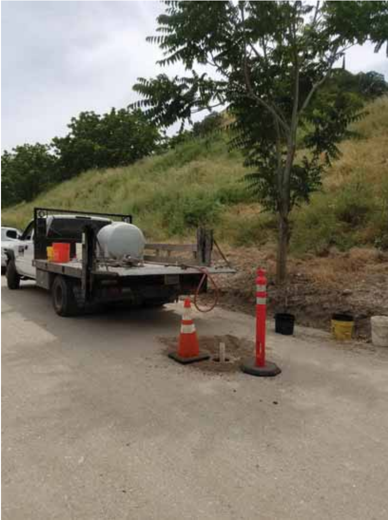
Infiltration test in progress
