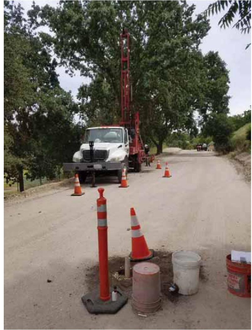
Infiltration test with drilling rig in background
