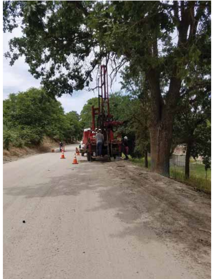
Boring an infiltration test pit at the shoulder of the road
