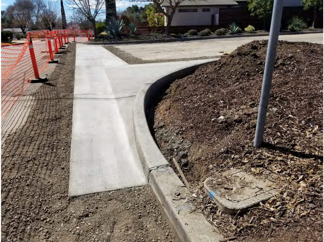
Completed concrete cross-gutter work at Tucker Avenue and Trigo Lane.
