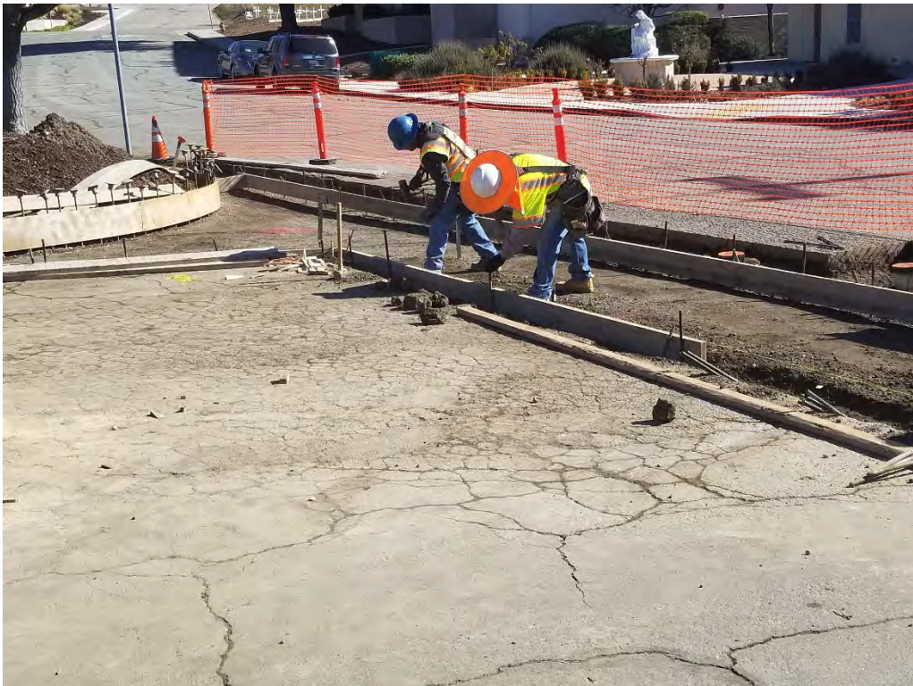
Construction of the concrete cross-gutter work.
