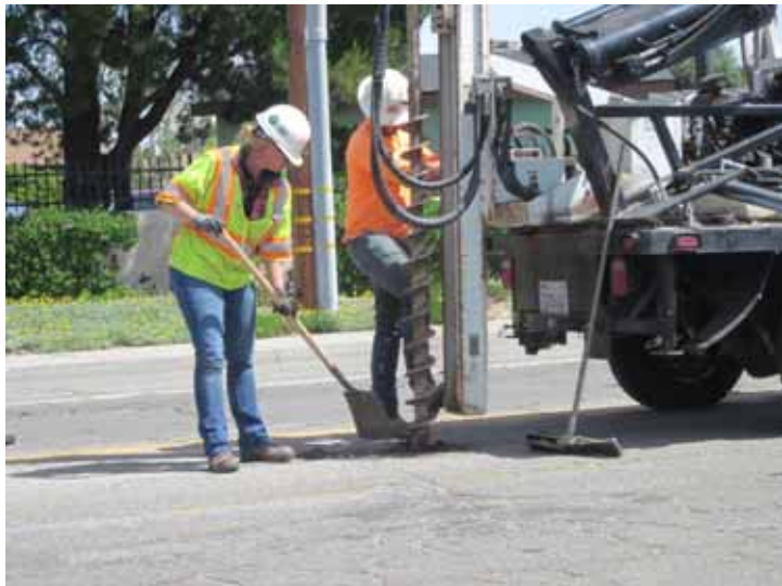
Boring Sherwood Road to obtain existing soils data to be used for the final design of the Road construction (04/24/2017)
