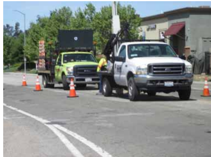
Boring Sherwood Road to obtain existing soils data to be used for the final design of the Road construction (04/24/2017)
