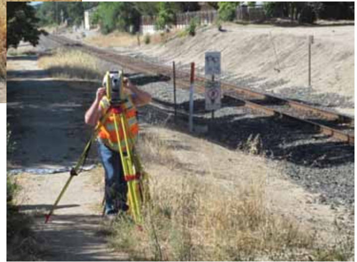
24 th Street Bridge Re-construction is underway. Surveyors are onsite to gather field data to be used for design (5/19/2017)
