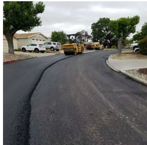
Surface Course (left) and Leveling Course (right)
