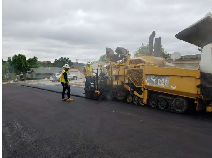
Paving the Final Surface on Trigo Lane
