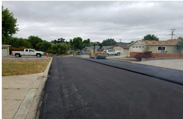
Leveling Course (left) and Surface Course (right)
