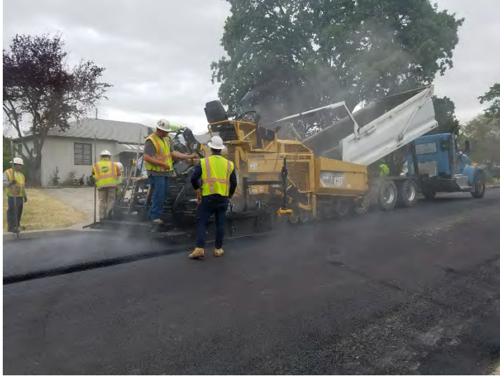
Paving the Final Surface on Trigo Lane
